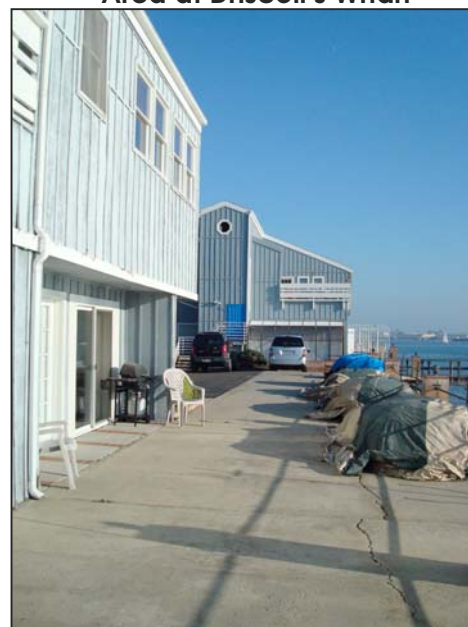
Figure 4-1 Footpath and Work Area at Driscoll's Wharf
