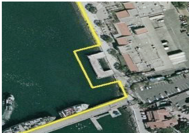
Fig 3.18 – Location of offloading cranes in Tuna Harbor
